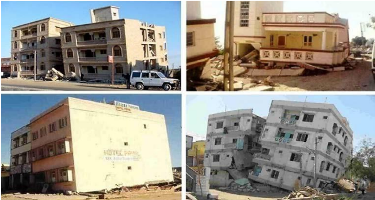
Figure 1. Earthquake damage due to soft story irregularity [17, 18].
